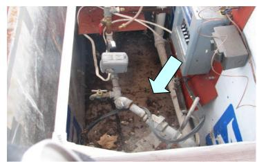
6. Take water sample from interior sample spigot (follow proper sampling taking procedures).
