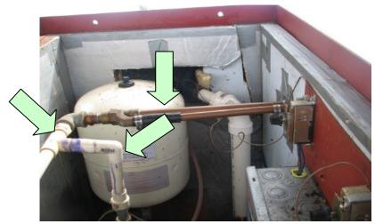
6. Open air valve on pressure tank.
