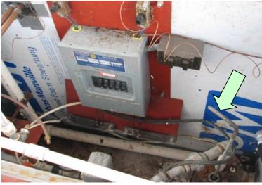
3. Open up test spigot to drain.
