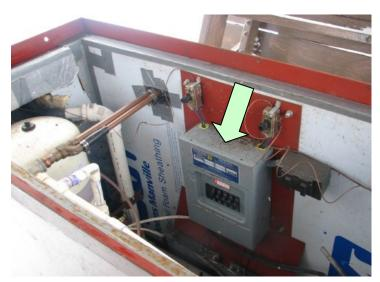
2. Open up drainage valve to allow water to drain back down to aquifer level.
