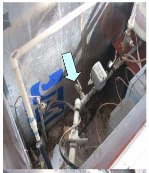
7. Shut down pump, replace cover and lock.
